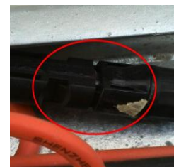
The cable is loose
